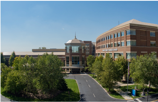
Miami Valley Hospital South
